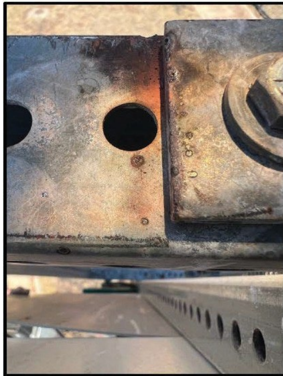
Figure 46. IMG_1816, 187721_765749- Speed sign arc melting
