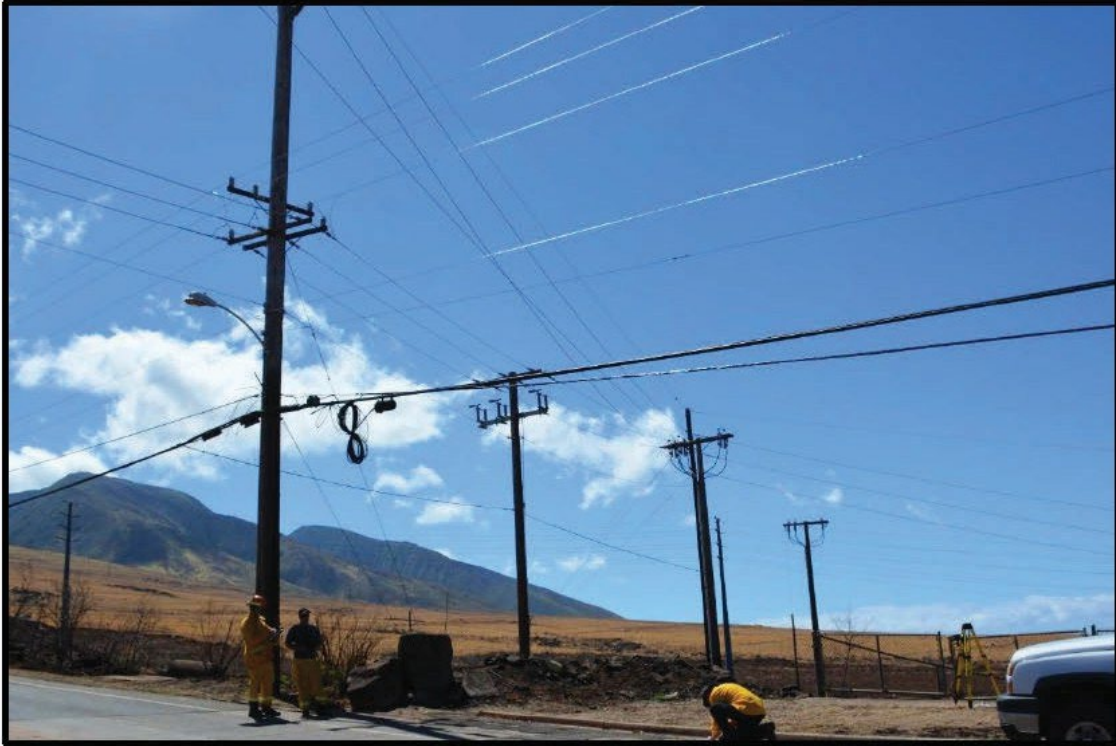
Figure 33. Lahaina, 187721_744901-Near Utility Pole 25 looking South
