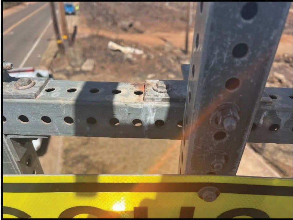
Figure 45. IMG_1812, 187721_765748 - Speed sign air-arc melting
