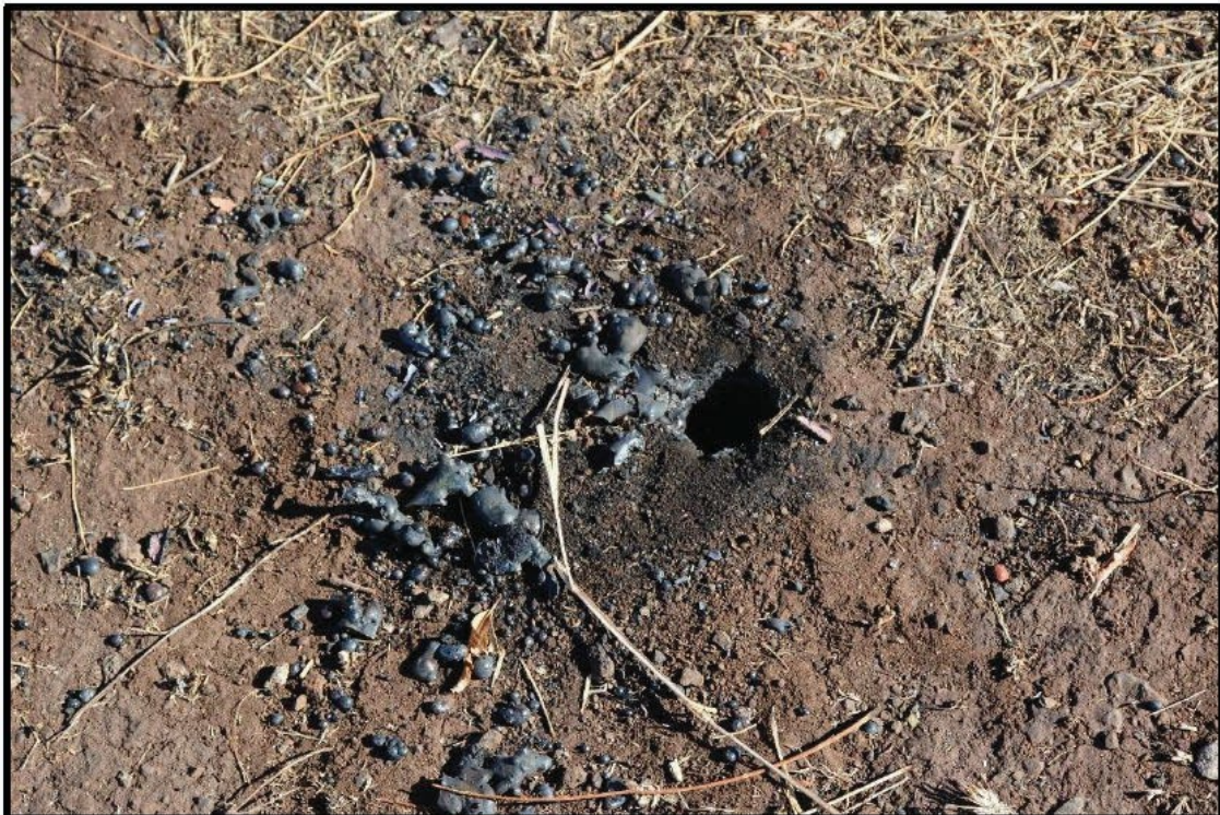
Figure 40. Lahaina, 187721_744759 -Fulgurites and molten metallic material between Utility Pole 24 and 25
