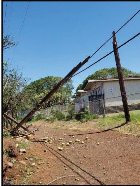
Figure 19. W-2 photo of Lahaina Snapped Pole 7A, 187721_763291
