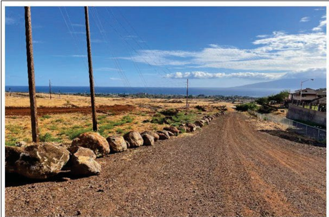
Figure 9 – View of the road put in post-fire (August 1, 2024)
