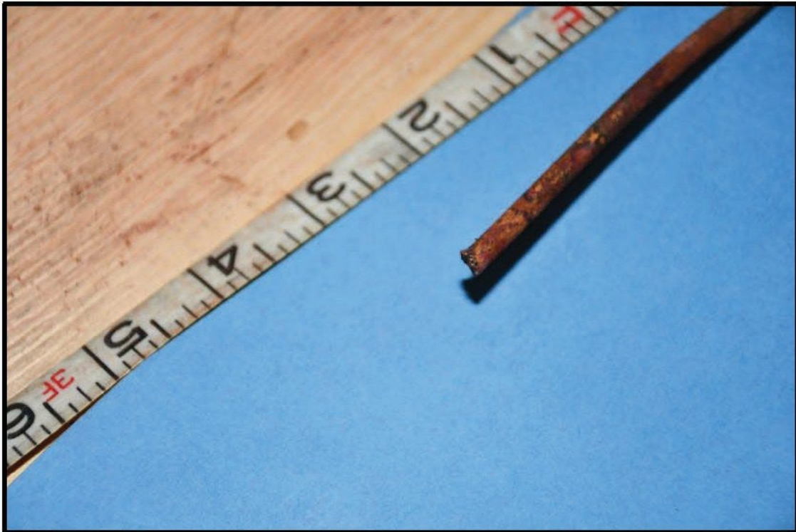
Figure 67. 187721_739528 -Lahaina DB#1 Loose Components
