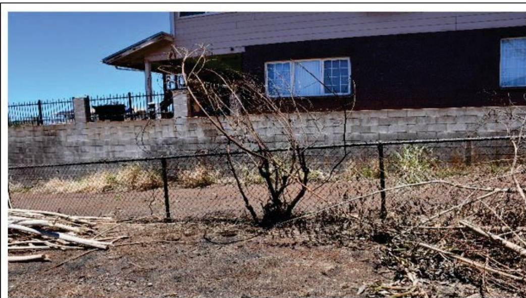
Figure 59 – Example of shrub growing into the chain link fence
