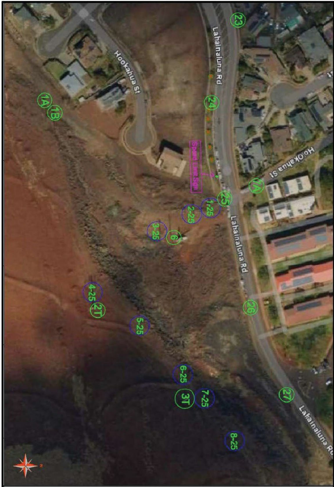
Figure 15. Lahainaluna Road Overall, 187721_765745 -Pole locations
