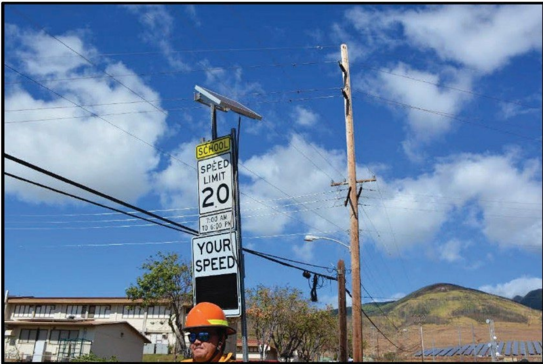
Figure 34. Lahaina, 187721_744922-Near Utility Pole 25 looking at overhead conductors and speed sign
