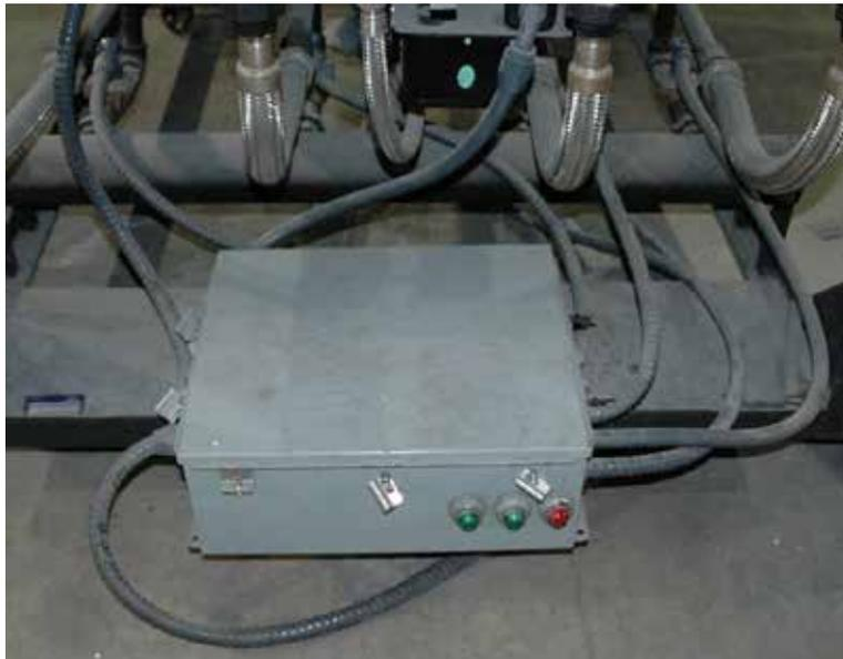
**Figure 12 - Gas burner electrical circuit box with LED indicator lights**
