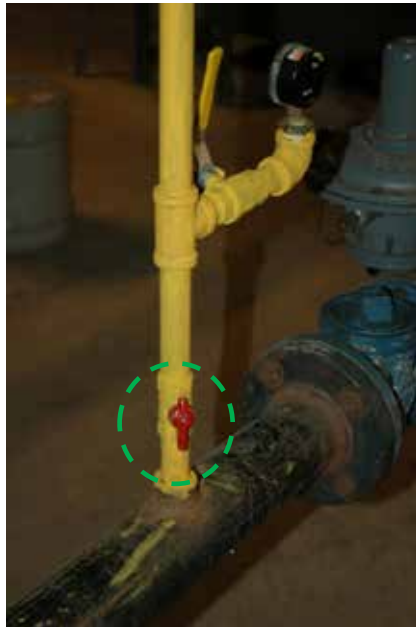
Figure 2. Combustion Calorimeter Connection to the Natural Gas Supply Line; Red Valve Shown in the “ON” Position.
