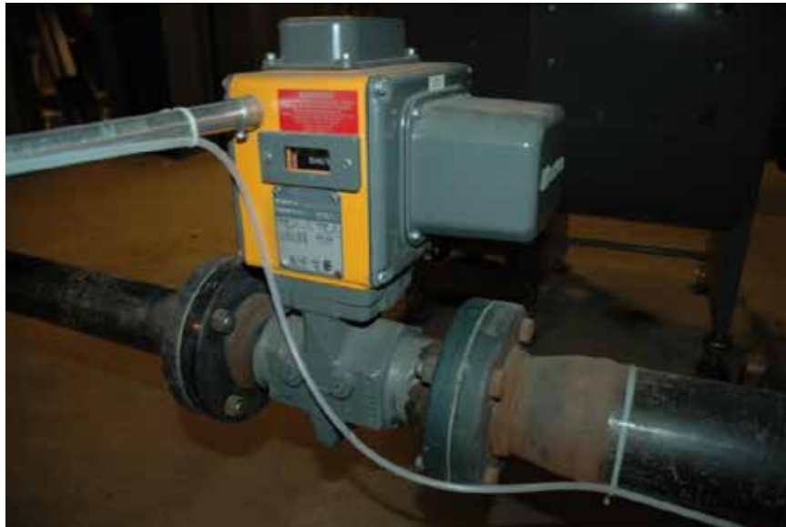
Figure 4 – Maxon Emergency Shutoff Valve
