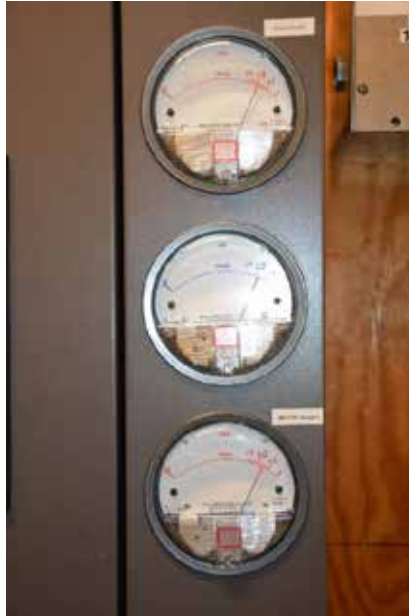
Figure 5. Combustion Calorimeter Pressure Gauges.
