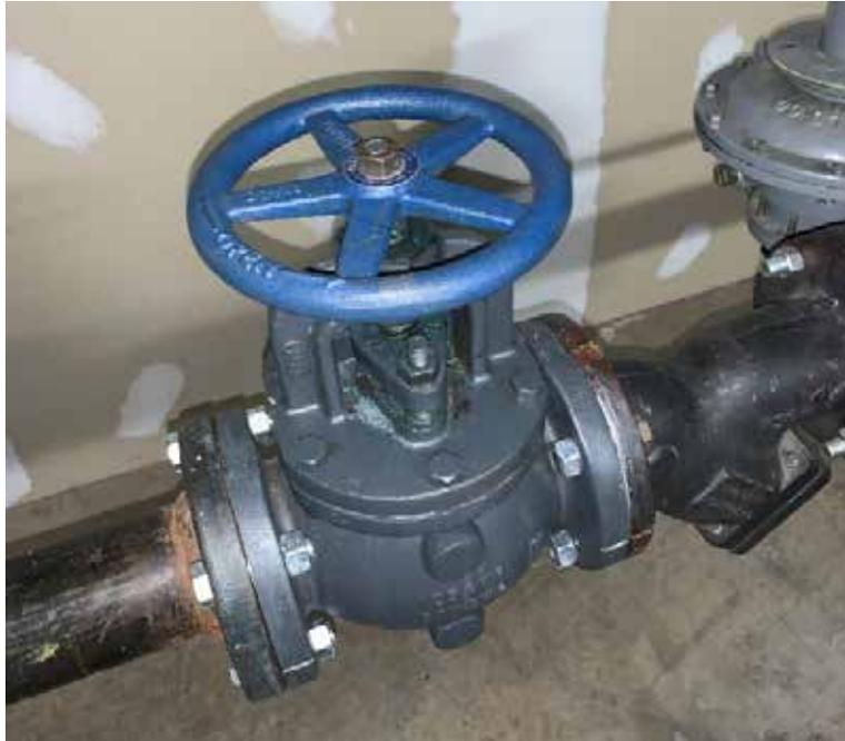
**Figure 2 –Manual Shutoff Valve for Mezzanine Gas Train**
