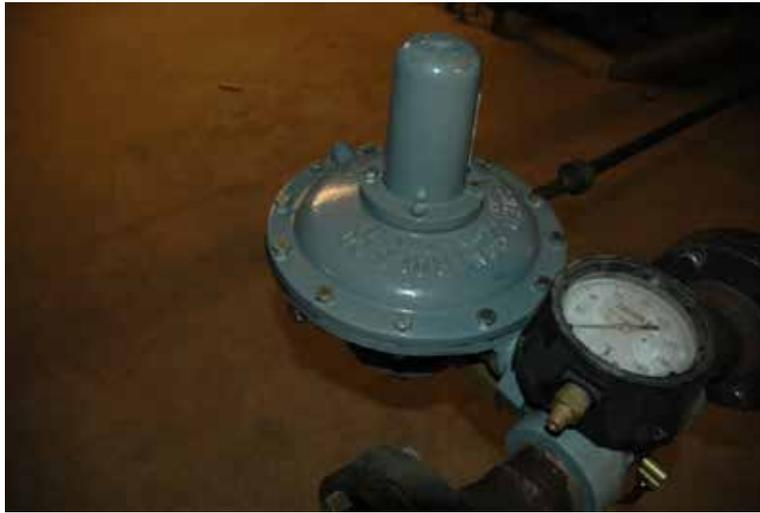
**Figure 3 – Type 99 Pressure Reducing Regulator**
