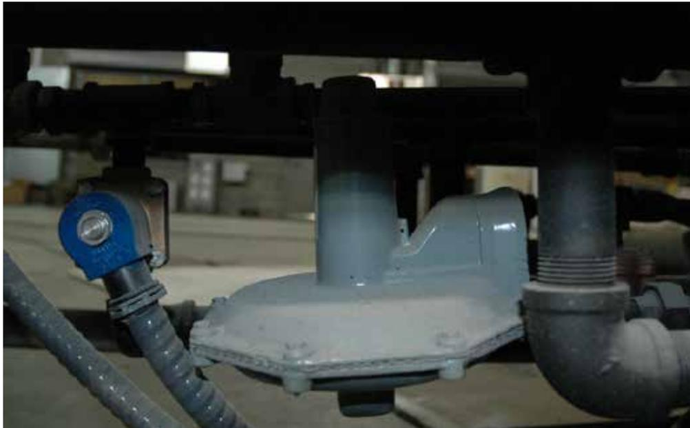
**Figure 10 – Pressure regulator (center) and solenoid valve (left) for gas burner pilot tube**
