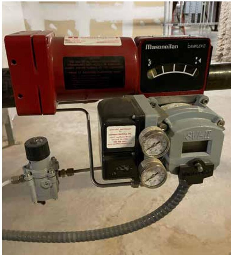
**Figure 7 – Masoneilan Flow Control Valve**
