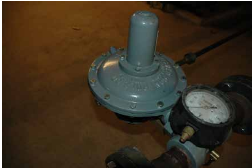
Figure 3 – Type 99 Pressure Reducing Regulator
