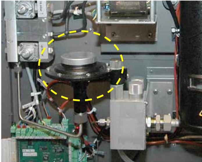
**Figure 8. Combustion Calorimeter Internal Gas Sample Regulator.**
