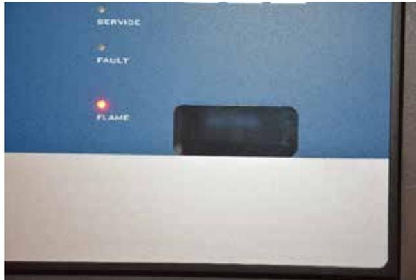
**Figure 4. Pilot Flame Indicator Light and View Port.**
