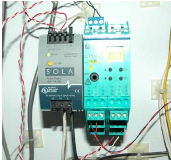
Figure 6 – Pepperl+Fuchs KFD-UFC-1.D Universal Frequency Converter and SOLA 24 VDC power supply
