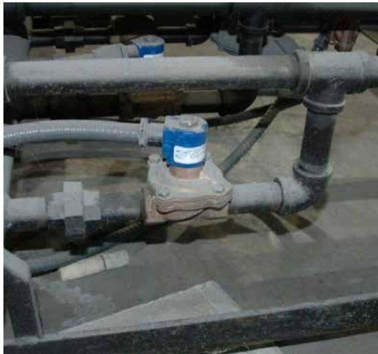
**Figure 9 – Solenoid valve connected to tube bank "4"**
