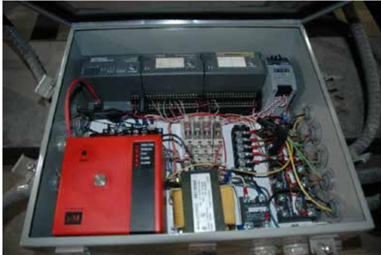
**Figure 11 – Gas burner electrical circuit box containing Fireye (bottom left corner), FieldPoint Module (top) and solid state relays (right)**
