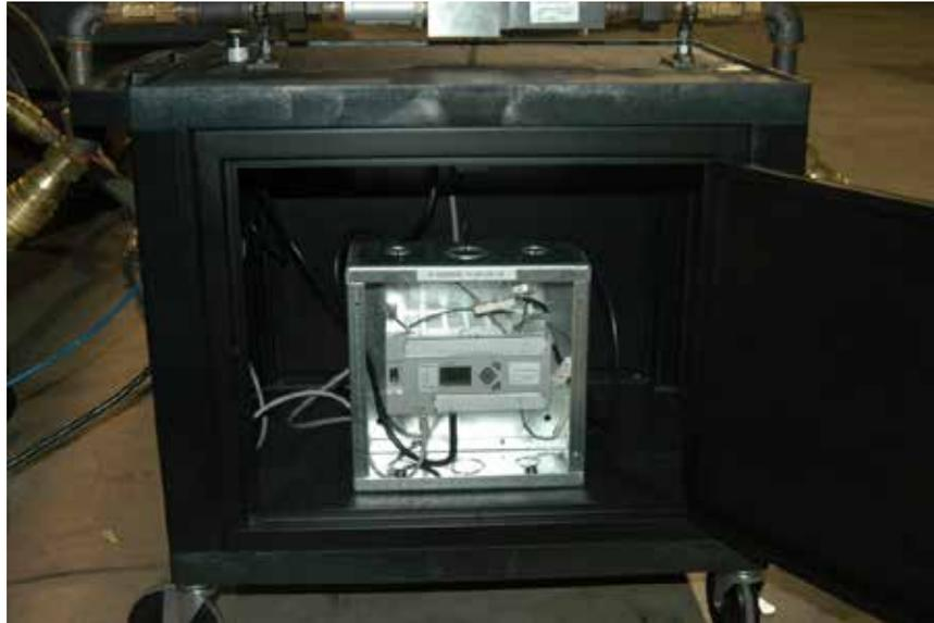
**Figure 5. Allen Bradley MicroLogix 1400 PLC inside Gas Cart**
