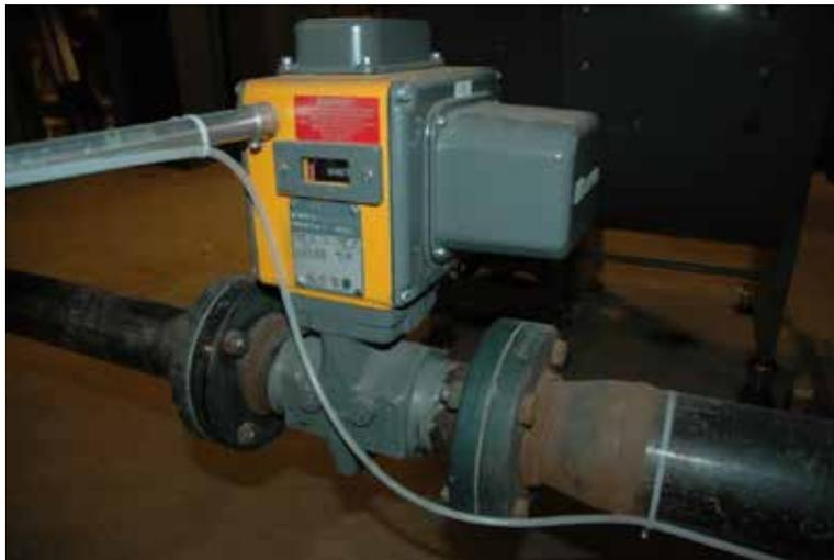
**Figure 4 – Maxon Emergency Shutoff Valve**
